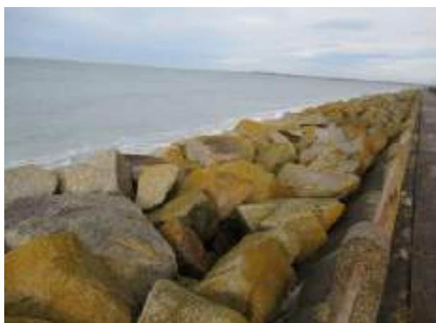
Figure 4: Digue Hauteville, source VTA 2019
